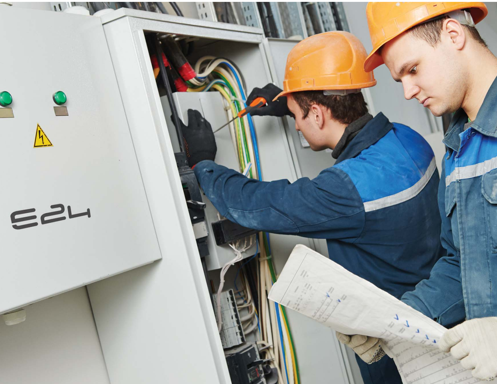
E24 technicians commissioning a new system.
